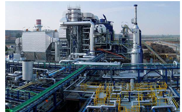
Biomass-CSP hybrid demo plant in Borges (Spain)
