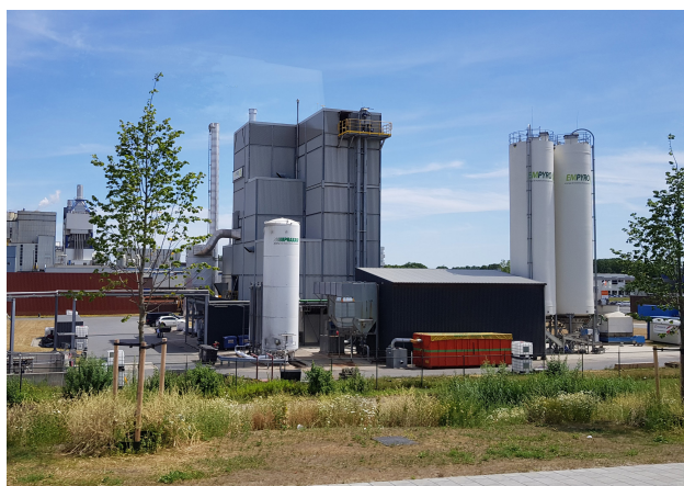
Figure 5: The Empyro pyrolysis plant in Hengelo (NL) Copyright: BTG BioLiquids
