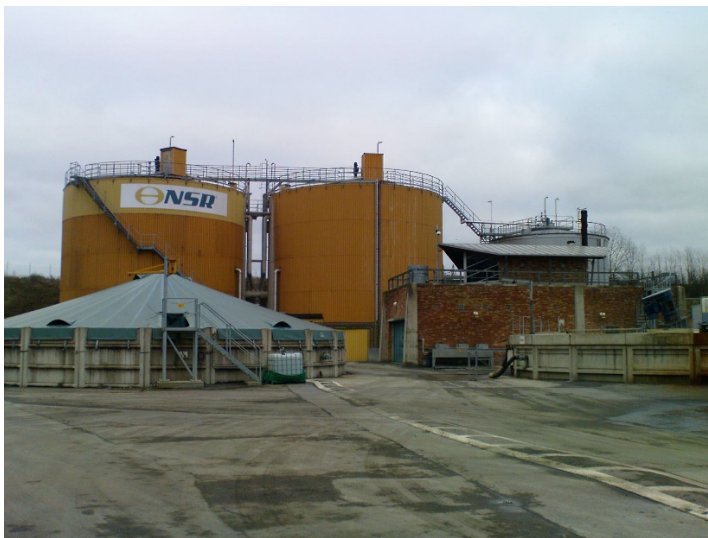
Continuous stirred-tank reactors (CSTR) have been used for a long time to digest different waste streams and produce biogas which can be upgraded to biomethane. Here two CSTRs are used to digest organic household waste and different industrial waste streams. Credit: Daniel Tamm
