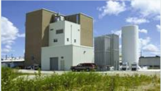
Gas Technology Institute, Des Plaines, Illinois, US
