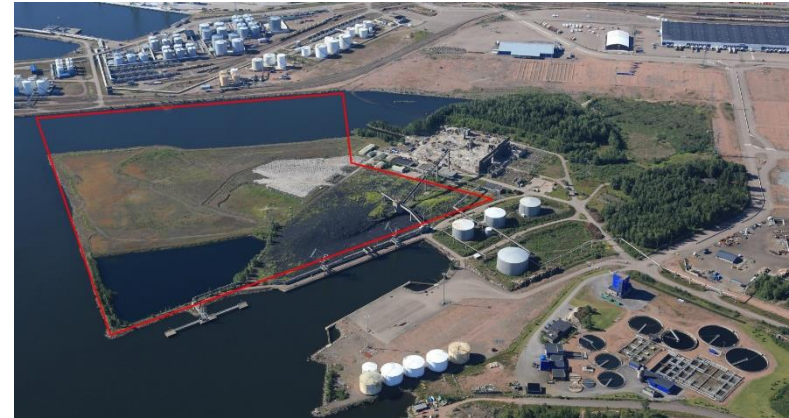
Kotka, Mussalo, Finland – the area of dismantled power plant formerly run by Pohjolan Voima
