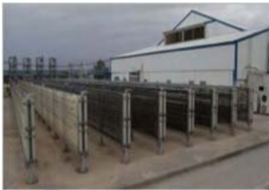
Figure 6: Fence –arranged tubular photobioreactors (Wilson (247) ).
