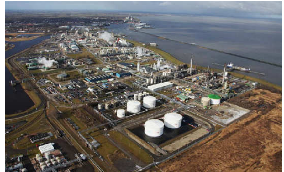
Site for the Woodspirit Plant
